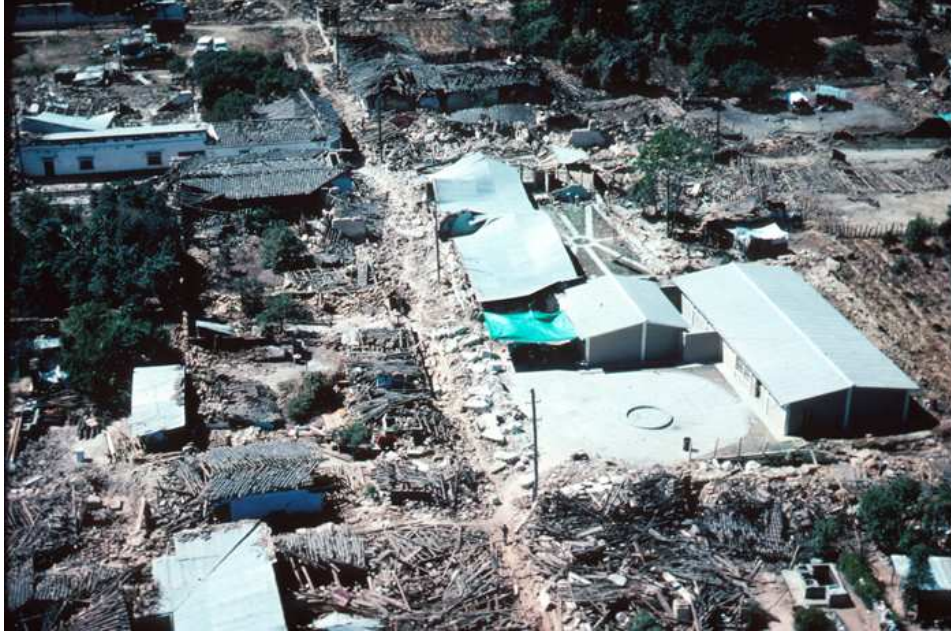
A typical highland village, located 33 kilometers northwest of Guatemala City that was devastated by the February 4 earthquake. Traditional adobe houses with tile roofs were almost completely destroyed, but the school buildings made of reinforced concrete block and corrugated asbestos roofs in the right part of this view are essentially undamaged. Source: slide 42, U.S. Geological Survey Open-File Report 77-165.
