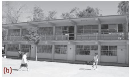
This structural model consists of a two-storey building with a footprint of 10 m × 40 m and a storey height of 3 m. The structure, the frame of which is shown in Figure 17.2(a), is divided into eight bays with a width of 5 m in the long direction and one bay with a width of 10 m in the short direction. A 2 m cantilevered slab on each floor acts as an access corridor for the different classrooms.
